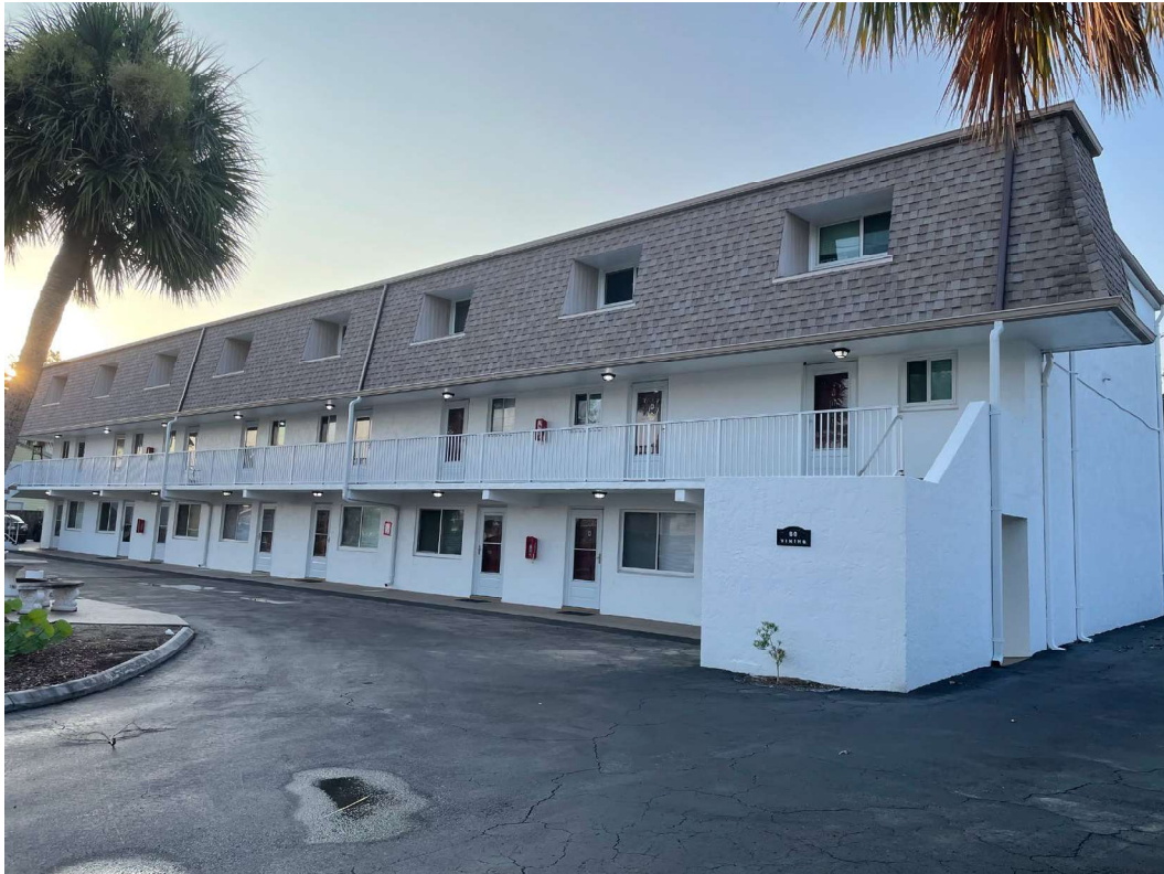
Photograph #1: Front elevation of building
