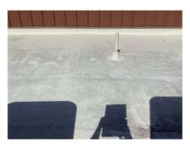
Data gathered from within the local market suggests a probable life cycle in the 18-20-year range for a professionally designed, installed and maintained roof including gutters. The current cost estimate includes removal and disposal of the existing roofing, typical minor repairs to the underlying roof structures, flashing, etc., and installation of like roofing.
