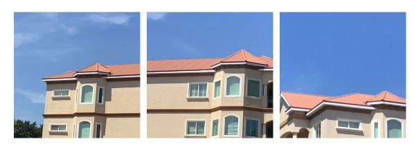
Data gathered from within the local market suggests a probable life cycle in the 25-30-year range for a professionally designed, installed and maintained roof including gutters. The current cost estimate includes removal and disposal of the existing roofing, typical minor repairs to the underlying roof structures, flashing, etc., and installation of like roofing.
